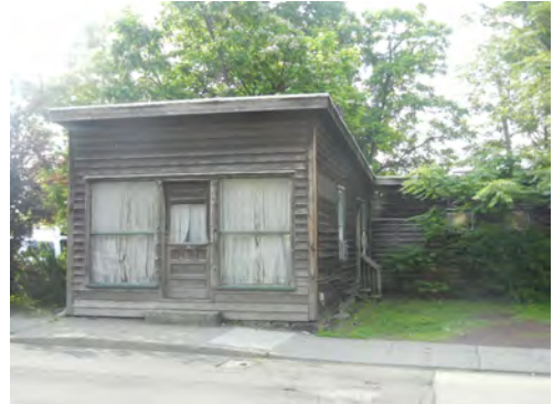
Existing Conditions at Wayne Ave
