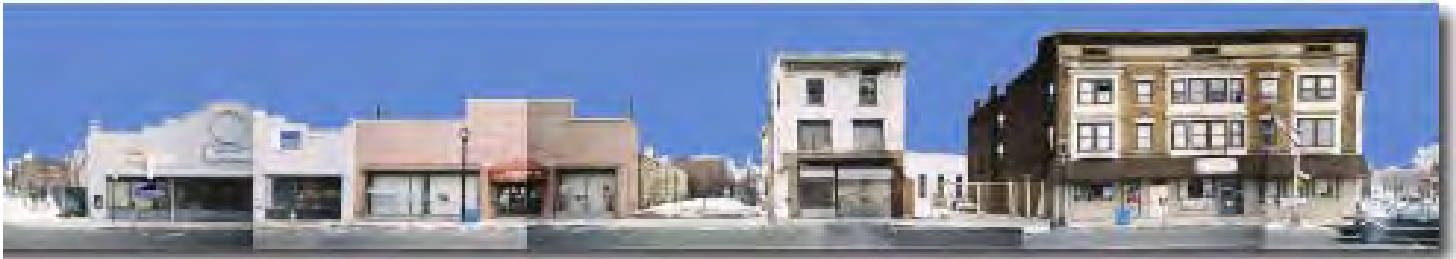
Existing Façade Study
